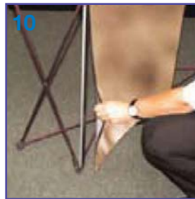
10 Smooth the graphic onto the mag bars, ensuring that it sits flat and is aligned to the centre line of each mag bar.
